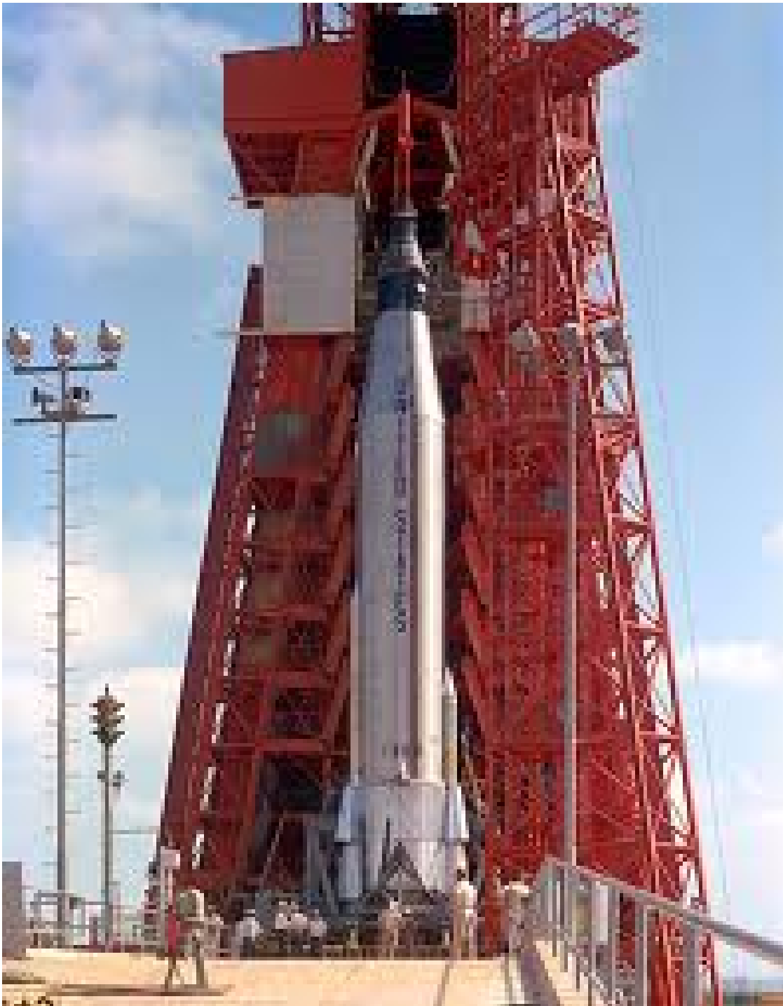
Figure 5: Atlas Missile Test Stand Service Tower
